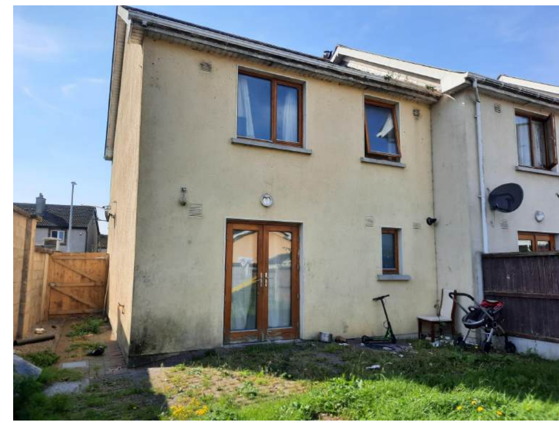
Photograph of existing Rear Elevation
