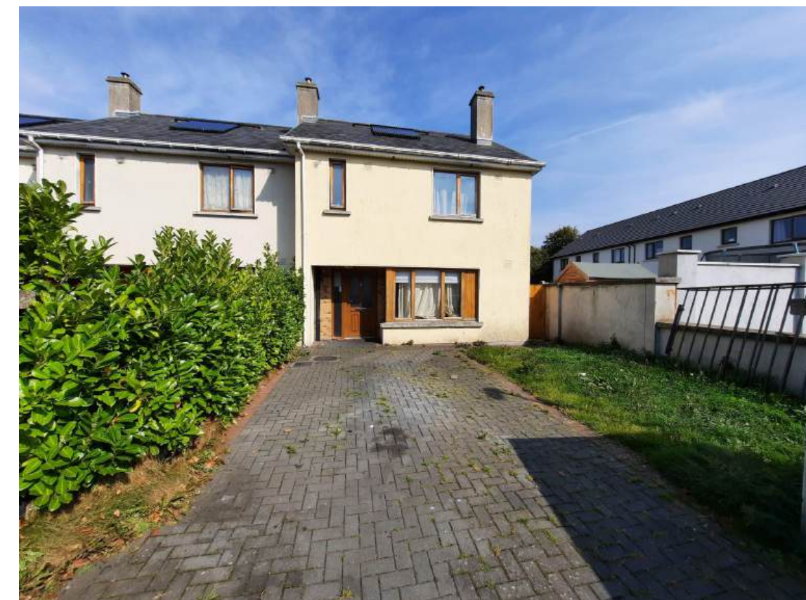
Photograph of existing Front Elevation
